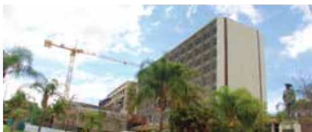
City Head Office during the construction stages.
